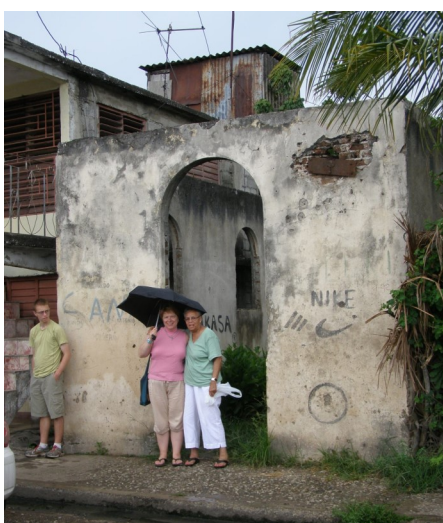
The exterior of the ruins of the St. John the Baptist Church.
